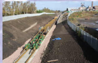
Laying new track at Newtongrange
